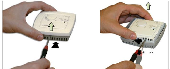
The bottom plate with terminals has a number of fixing hole combinations. Select suitable holes and screw the bottom plate onto the wall or connection box, so that the arrows on the bottom plate point upwards. Do not tighten the screws too hard! With surface-mounted cabling, break out suitable holes from the marks in the plastic.
