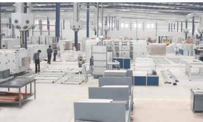
Manufacturing Facility, India.
