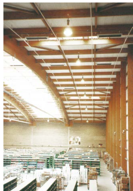
Radiant heaters are especially profitable in buildings with high ceilings as no heat losses occur between the heater and the floor.
