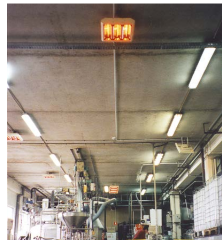
IRCFC is often installed in large warehouses. They give instant and effective heat which make them profitable quickly.
