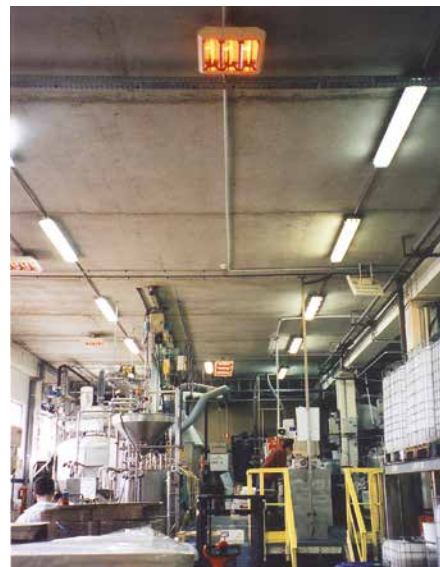
IRCF is often installed in large warehouses. They give instant and effective heat which make them profitable quickly.
