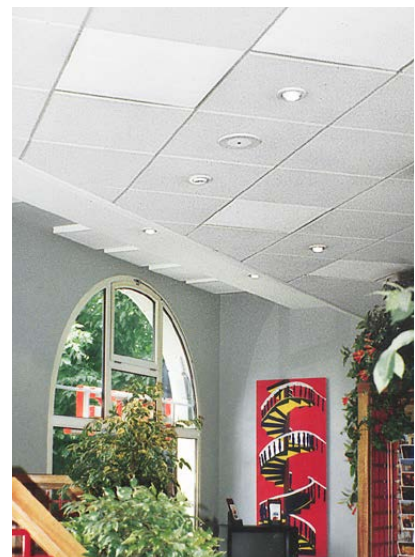
By putting the heater in the ceiling, valuable wall and floor space is saved.
