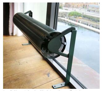
Installed by a window the ribbed pipe radiators effectively counteract cold draughts that frequently form by large glazed areas.
