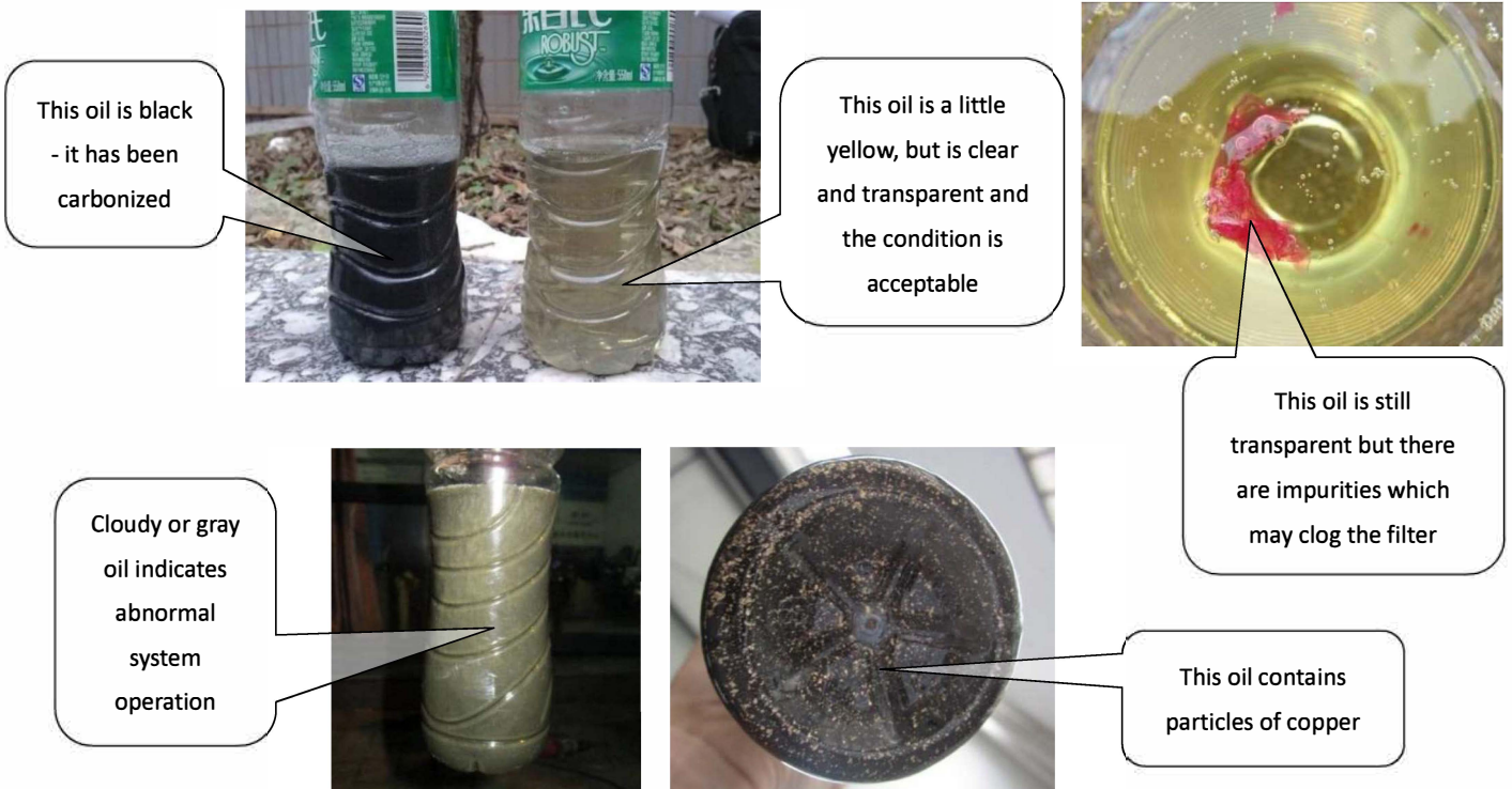
Figure 6-2.10: Inspecting compressor oil
